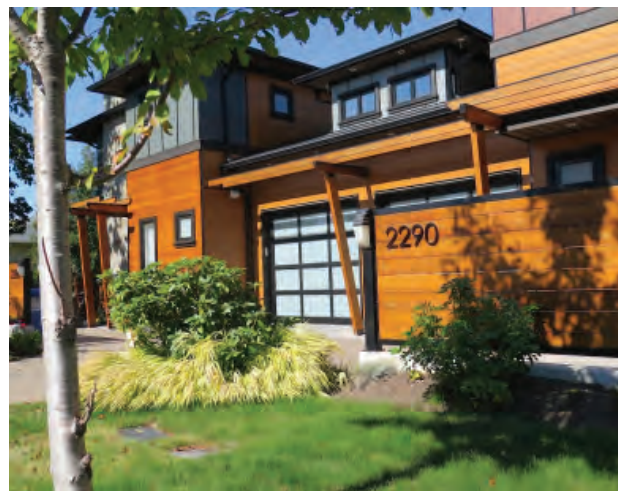
Example of a duplex with significant façade articulation (guideline 13), and high-quality siding (guideline 14).
