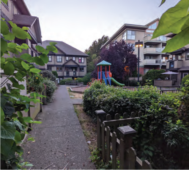
Example of a central common outdoor amenity space (guideline 77), with easy pedestrian access to individual units, where possible (guideline 77 c).
